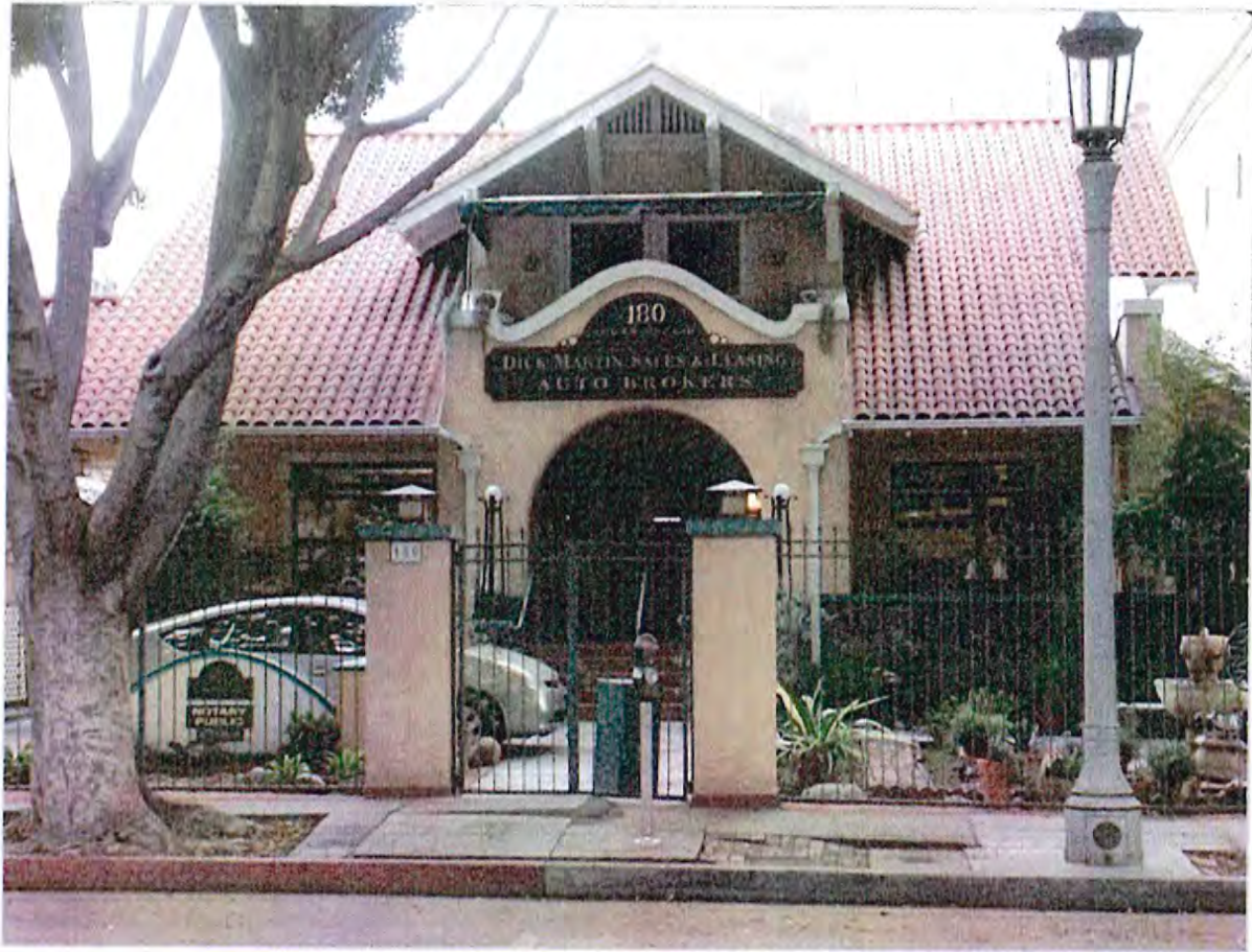
Figure 2: West Elevation. Source: GPA, November 2013.
