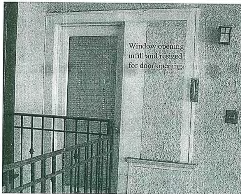
Figure 9. Looking north, south elevation of rear upper story, window opening infill and resized for door opening; 1994 alteration permit.
